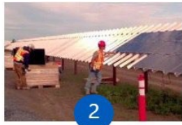
Panels installed on racking
