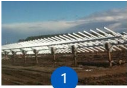
Racking mounted on piles
