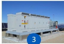
Inverter/Transformer Skid
