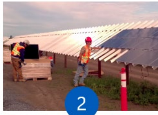
2 Panels installed on racking
