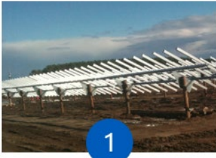
1 Racking mounted on piles
