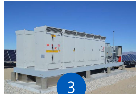
Inverter/Transformer Skid
