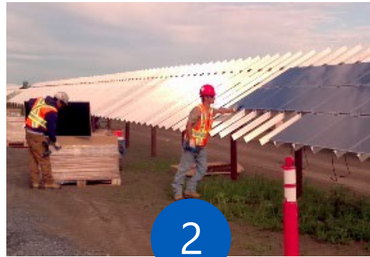
Panels installed on racking
