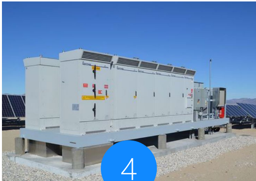
4 Inverter/transformer skid
