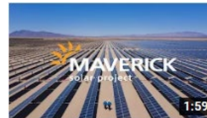
Maverick Solar Project
